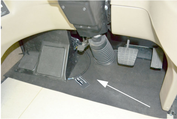
CB Power Wires -Typical View
