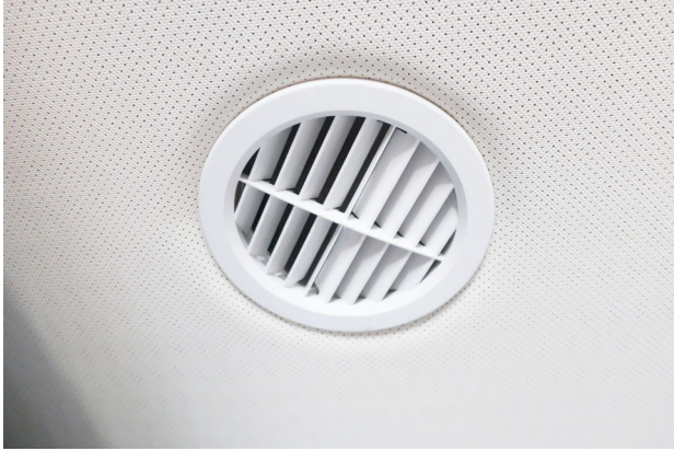
Return Air Vent (Grasp louvers and pull straight down to remove air vent) -Typical View
