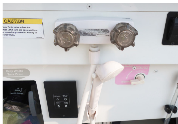
Exterior Shower/Wash Station –Typical View
