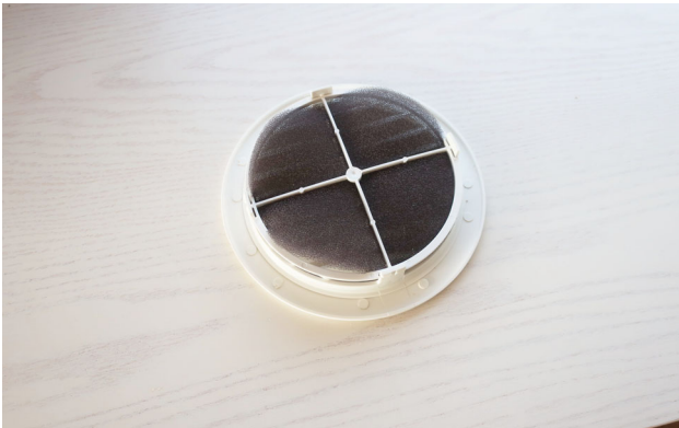
Air Filter (Located on back side of Return Air Vent) -Typical View
